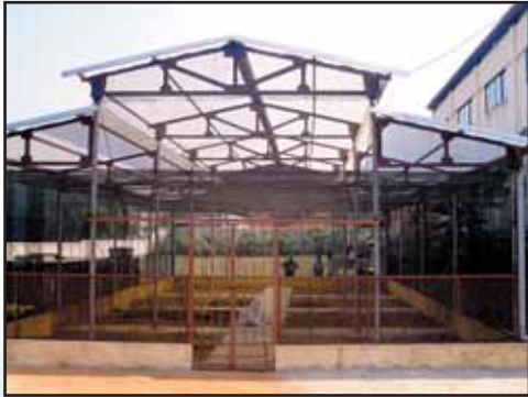
New green house for vocational practice
